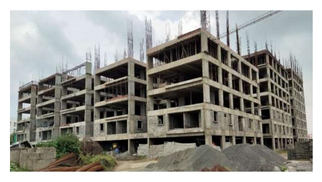
Block D1: Columns upto Third floor level 50% completed. Shuttering & Barbending works for 1<sup>st</sup> half of Third floor level 25% completed.
