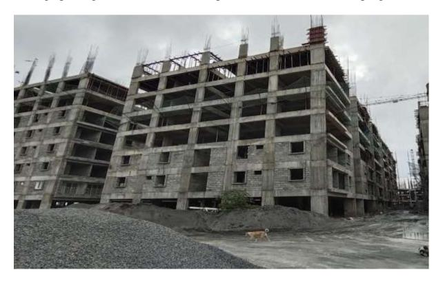
Block C3: Columns upto Sixth Floor Level 50% completed. Shuttering and barbending work for 1<sup>st</sup> half of Sixth floor level 15% completed.
