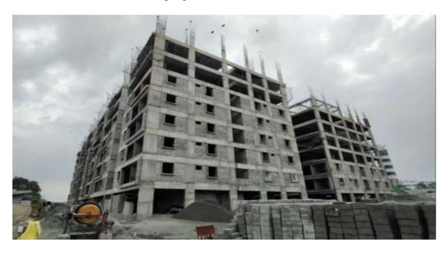
Block C2: Seventh Floor level slab concrete casting 100% completed. Column casting upto Eight floor level 15% completed and balance work on progress.
