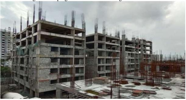
Block D3: Fifth floor level slab concrete casting 100% completed. Columns concrete work upto sixth floor level on progress.
